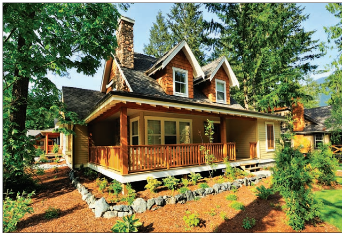
Shining opportunity: builders are ramping-up construction of units such as this cabin near Cultus Lake to meet buyer demand in advance of the HST's introduction in July
